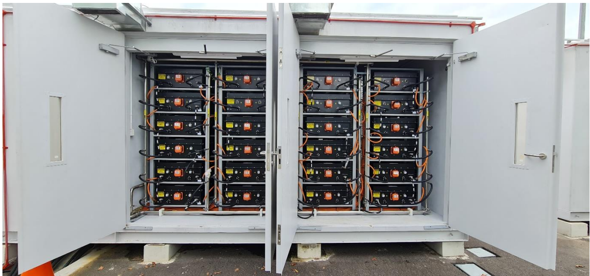
Battery Modules within the Battery Container
