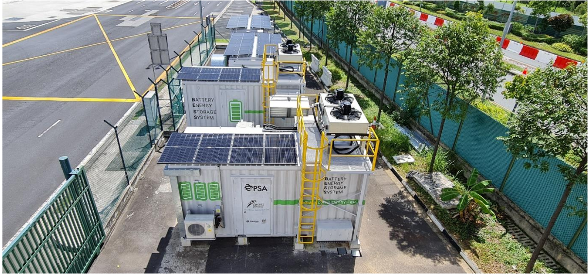
The setup consists of two Battery Containers and two Power Conversion System (PCS) containers.
